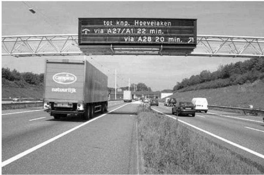
Figure 2.3: Route guidance in a modern freeway
